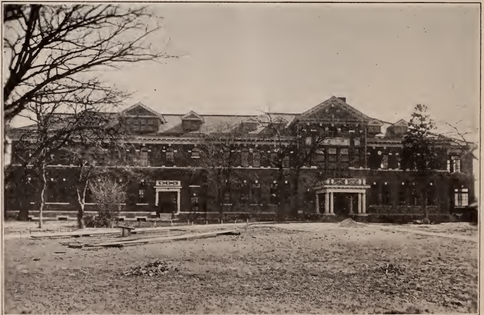
VORNHOLT MEMORIAL EXTENSION (AT LEFT), SECOND RECITATION HALL OF MIYAGI COLLEGE, SENDAI, JAPAN
